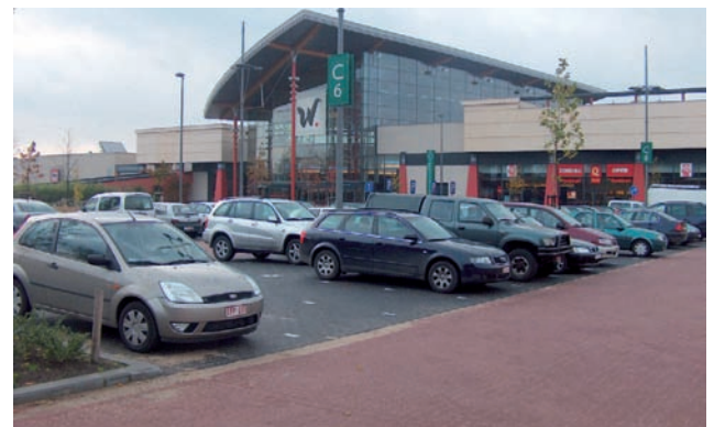
Parking pavement made with permeable paving blocks
